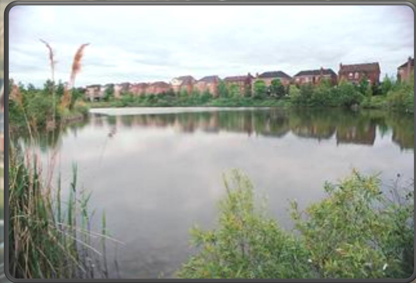
Stormwater management pond in a residential area
