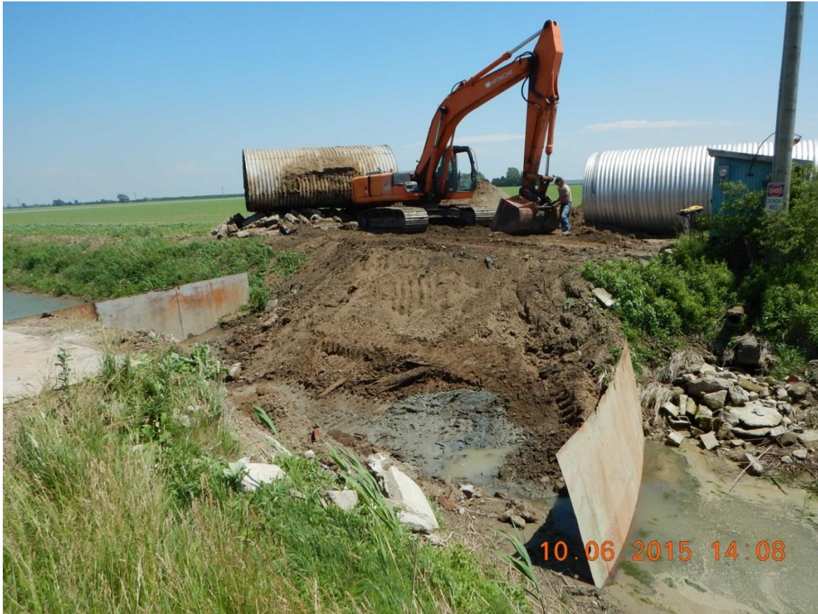
Figure 2. Isolation of Site
